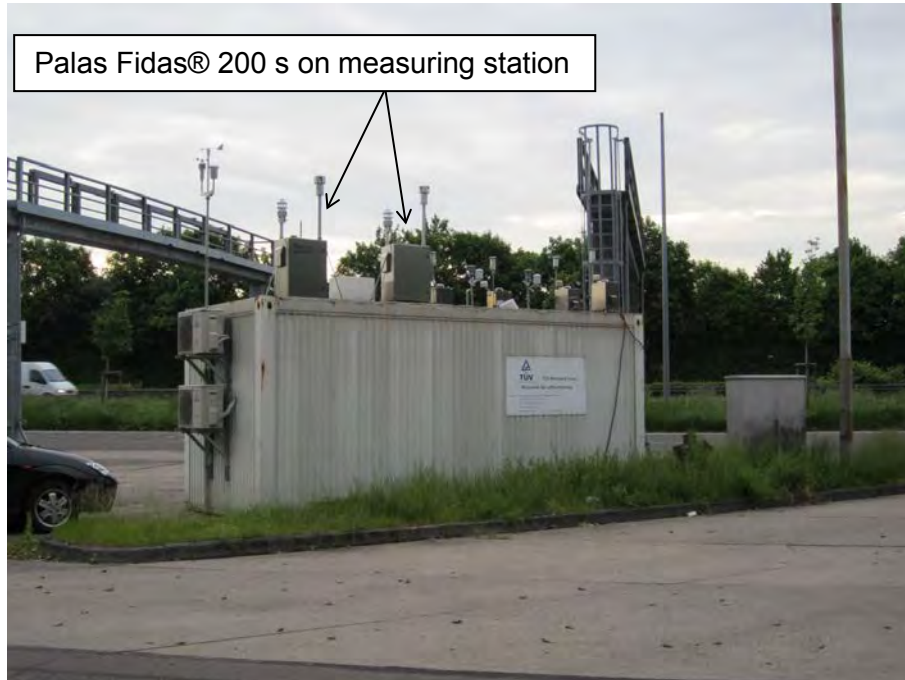
Figure 14: Fidas® 200 S measuring systems on measuring station
