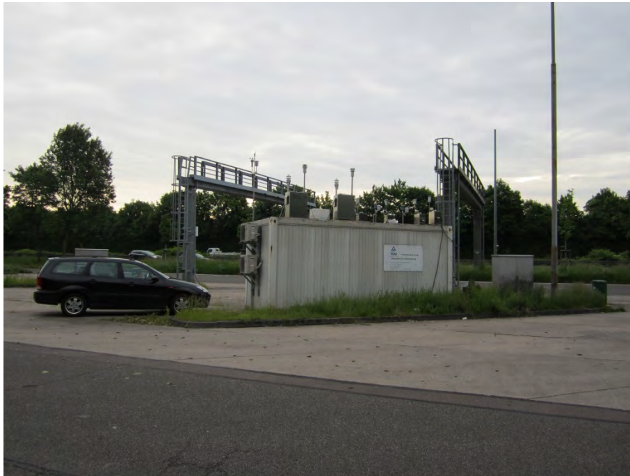
Figure 37: Field test site in Bornheim, summer
