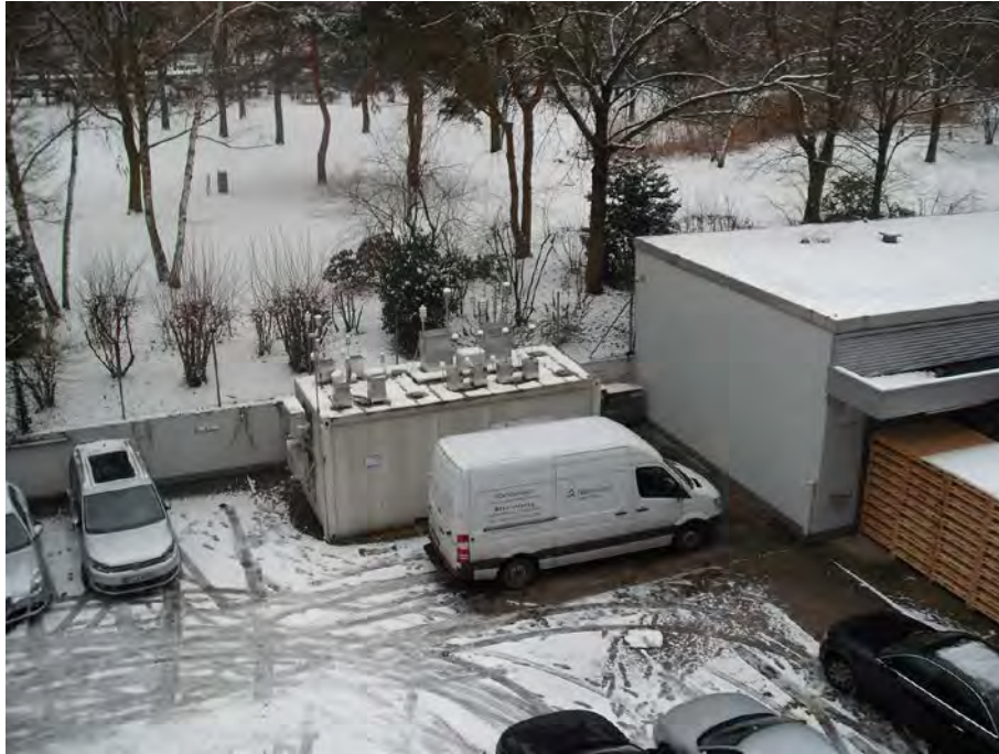
Figure 32: Field test site Cologne, summer & winter
