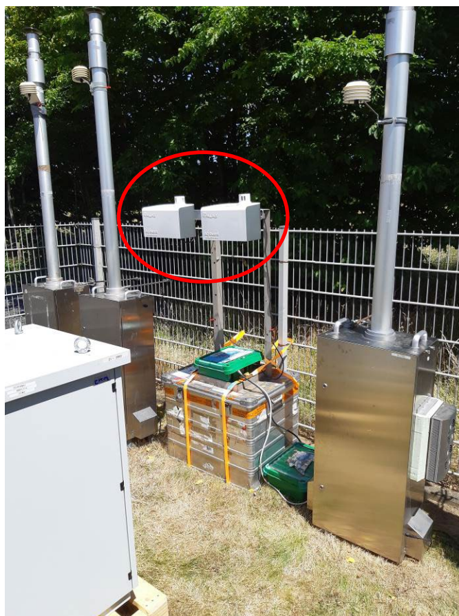
Figure 20: Field test site Niederzier (AMS in the middle)
